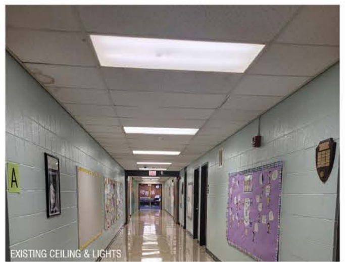
EXISTING CEILING & LIGHTS
