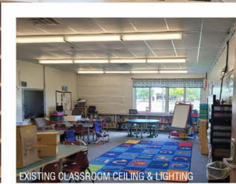
EXISTING CLASSROOM CEILING & LIGHTING
