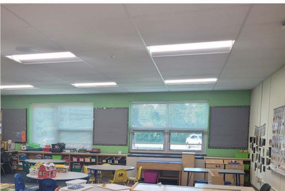
NEW CLASSROOM CEILING & LIGHTING
