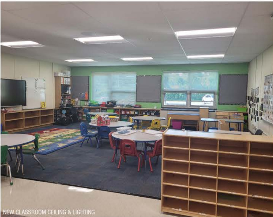
NEW CLASSROOM CEILING & LIGHTING
