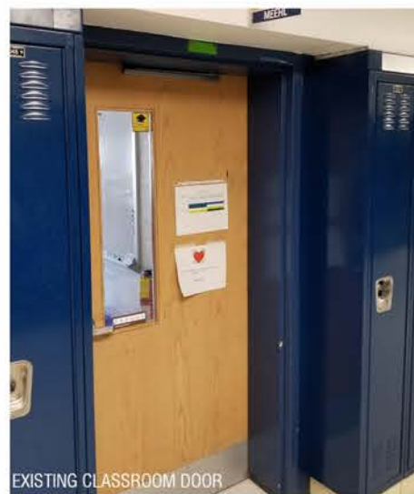
EXISTING CLASSROOM DOOR
