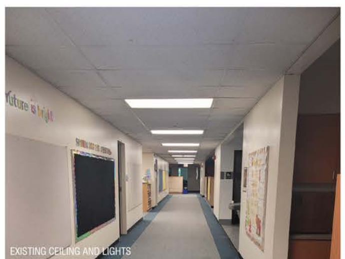
EXISTING CEILING AND LIGHTS
