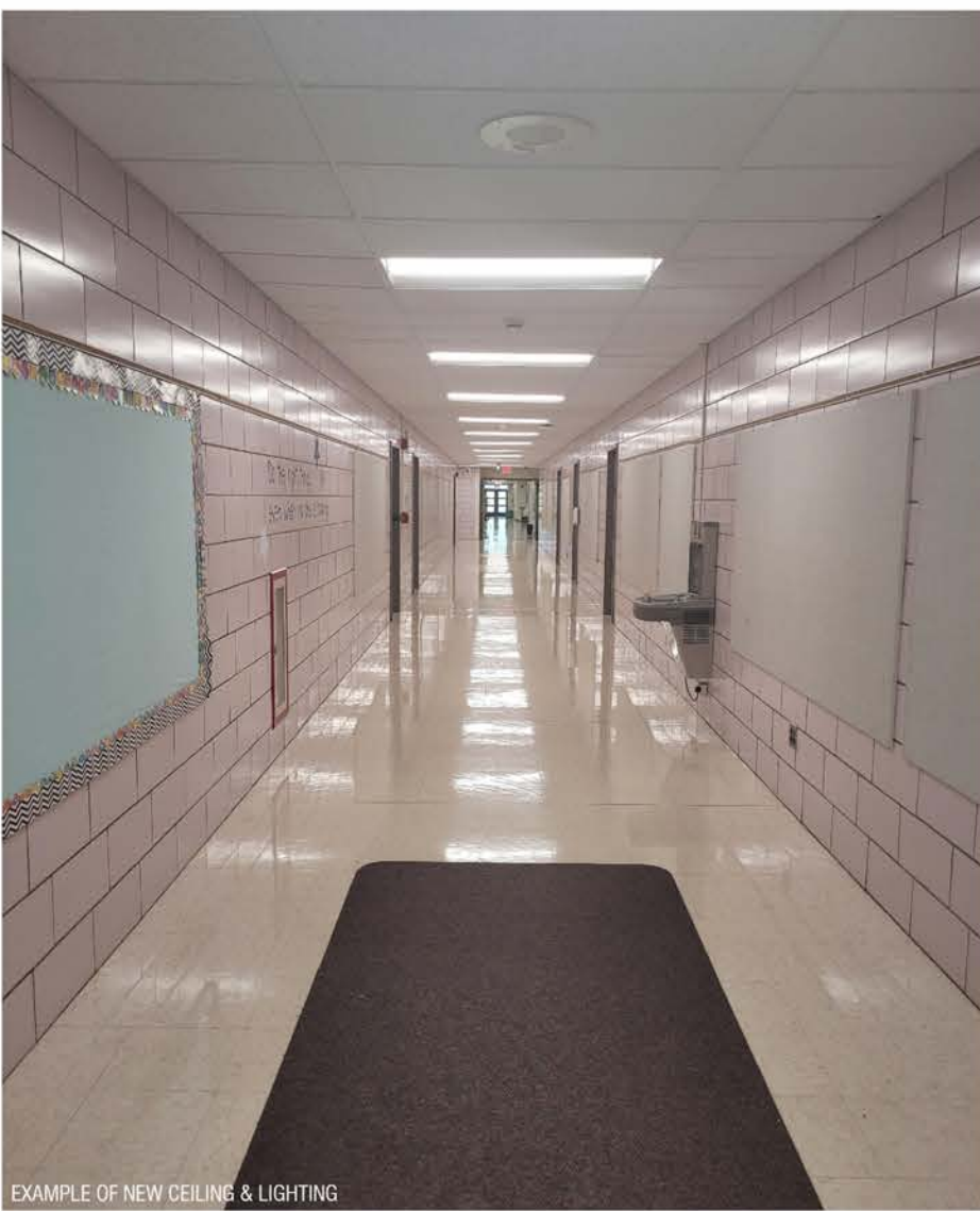
EXAMPLE OF NEW CEILING & LIGHTING
