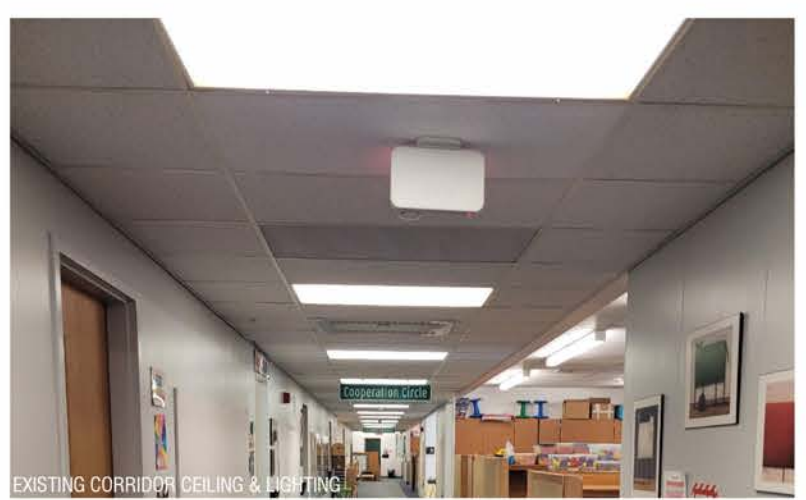
EXISTING CORRIDOR CEILING & LIGHTING
