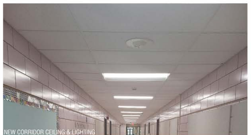
NEW CORRIDOR CEILING & LIGHTING
