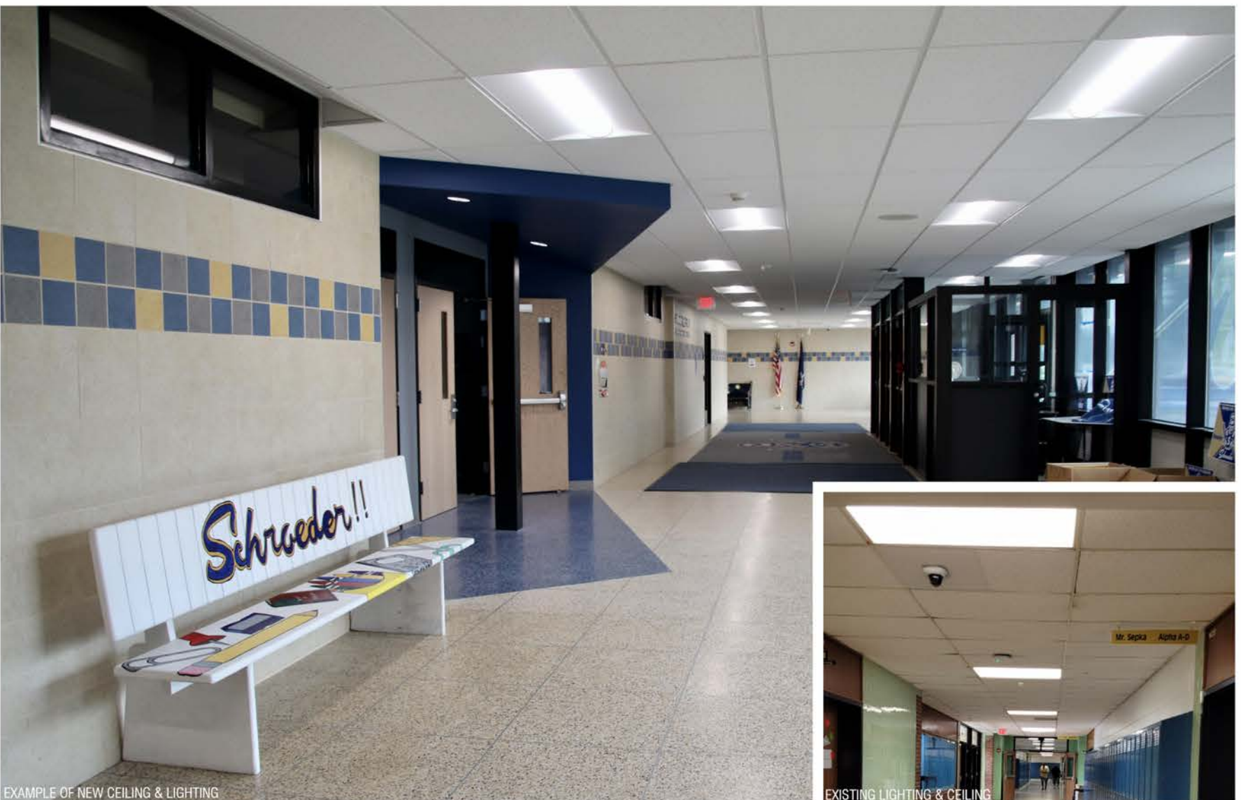
EXAMPLE OF NEW CEILING & LIGHTING
